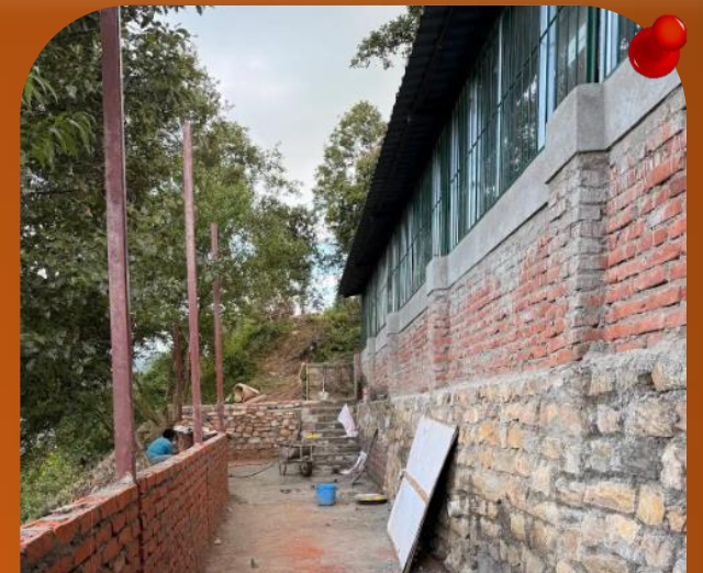
Civil structures under construction primarily for the development of the RenewHydro test setup at TTL
