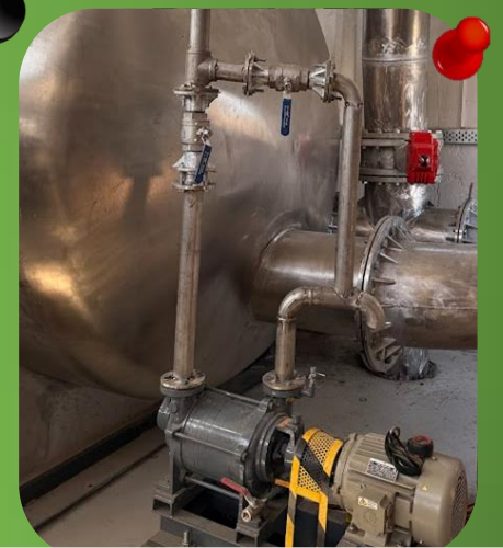
Installation works in the Low Pressure Tank of TTL
