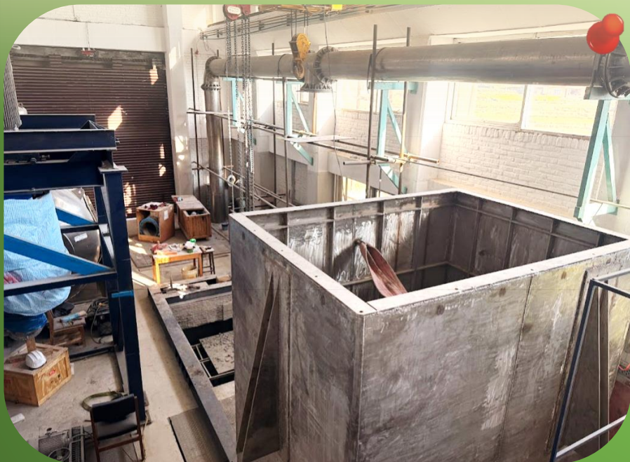
Installation of calibration tanks ongoing at TTL
