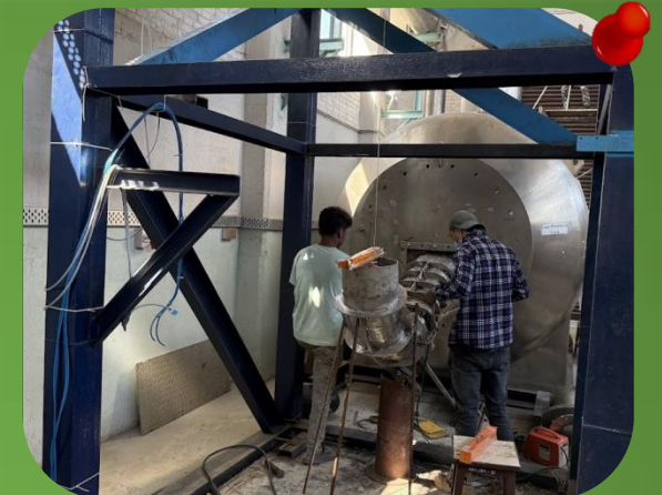
Installation of Draft tube in the Low Pressure Tank (Nov 19)
