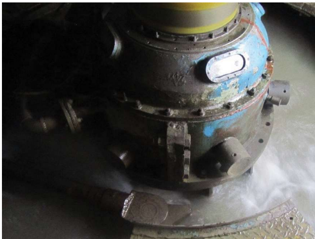
Fig. 1 Leakage of water from shaft seal during the operating condition.
